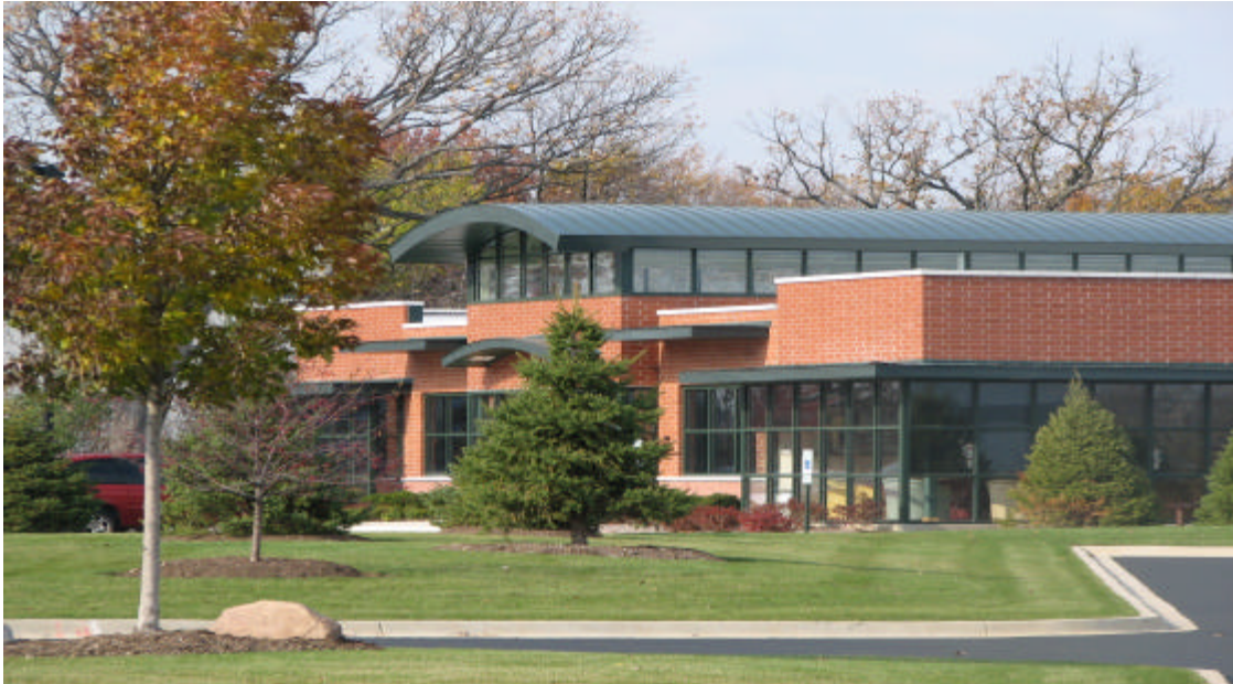
Becmar Sprinkler Company, Bridge Lane
