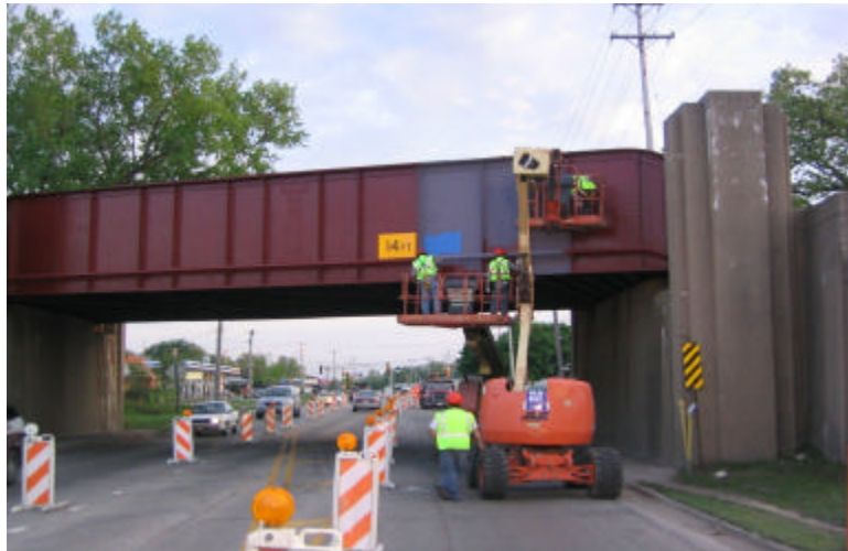
US Route 47 Railroad Overpass
