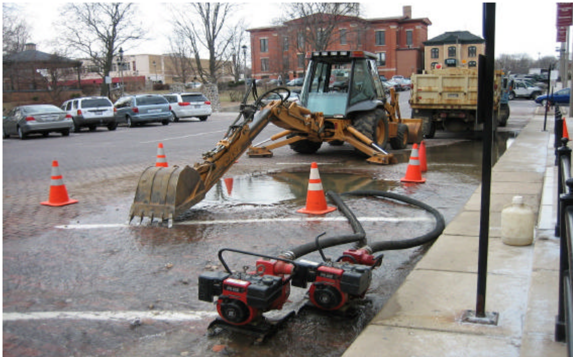
Water Main Repair, Cass Street
