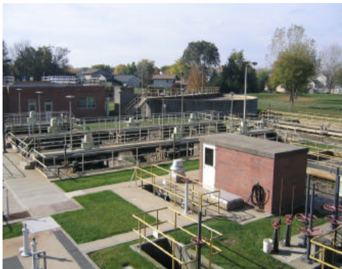
North Side Sewage Treatment Plant
